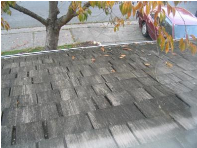
1.0 Picture 1 Cedar roof
