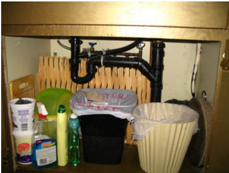
10.4 Picture 1 No garburator
